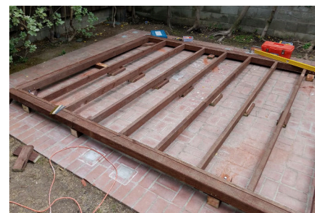
Wood Frame on Pre-Existing Slab
