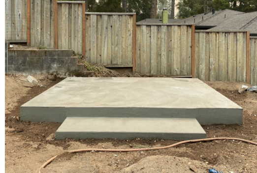
Concrete Slab on Grade (with optional step)
