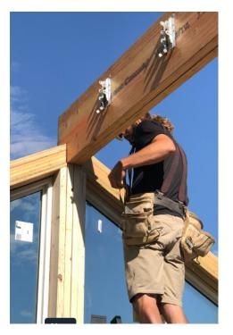
Once both ridge beam sections are in place, be sure to secure them together with construction screws. Typical pattern is three (3) screws at the mid-point between each rafter.
