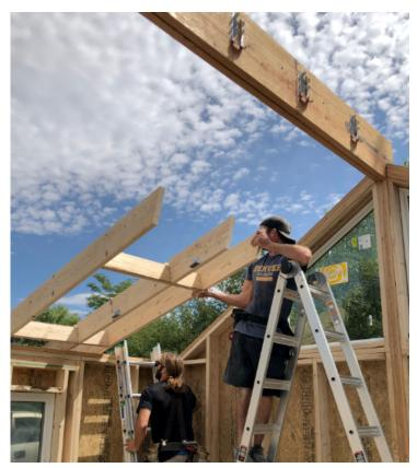
Guide each rafter section into place. You can run a screw through the top of rafter and into the ridge beam to secure it wall working. Install rafter hanger nails in pre-drilled holes to permanently secure the rafters to the ridge beam and walls.
