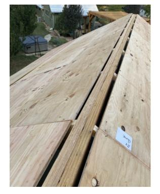
Sheathing should terminate below the ridge beam to allow for ventilation.
