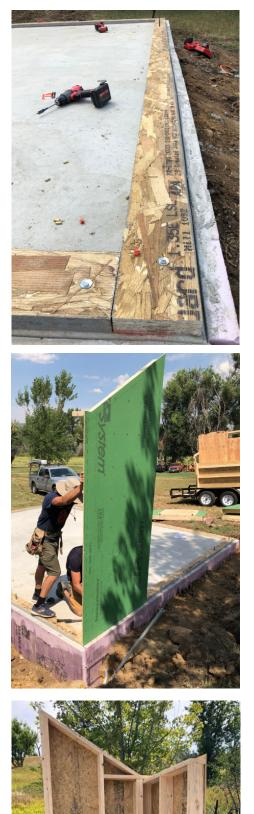
Pin sill plate to slab. Ideally, the sill plate is inset from edge of slab by 1/2" to allow wall sheathing to be flush with edge of slab.
