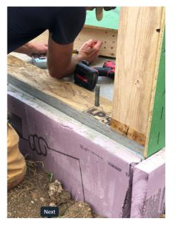
In some cases, hold-down embeds are called out. If this is the case, you will need to drill holes in the sill plate as well as in the bottom wall plate when you're standing wall panels. Carefully measure the center line of the embed, then use a 1" paddle bit to drill a hole for the embed to pass through.
