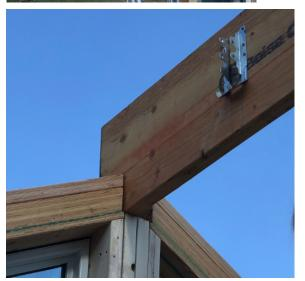
Whether the rafter hangers are pre-installed, or you install them in the field, ensure the bottom of rafter will be at the same elevation as the top of top plate on the wall.
