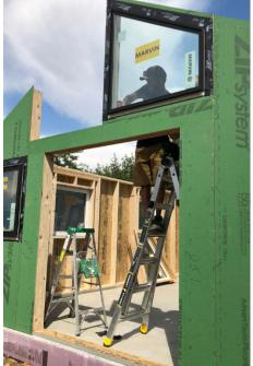
Carefully place trapezoid window panels on top of header. The top plate of the adjacent wall panel should be flush with the top of window header.
