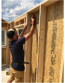
Install construction screws in a staggered 12" o.c. pattern at each panel-to-panel joint. 3" screws should be used where single studs meet. 5" screws should be used where a single and double stud meet.
