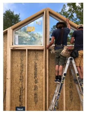
Installation of window panels at a back elevation. Ensure the edge of window header is flush or inset slightly (1/16") from the exterior edge of vertical stud, which will ensure the king stud will fit properly.
