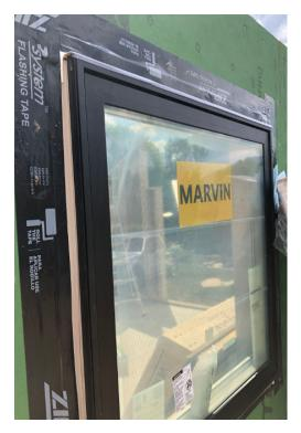
You may notice the windows installed in wall panels move when pushed. If this is the case, call Studio Shed as there is a procedure for installing screws through the window frame to secure the window.
