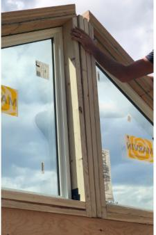
Carefully install remaining window panels. If necessary, temporarily screw the panel into adjacent studs to secure the window panel.
