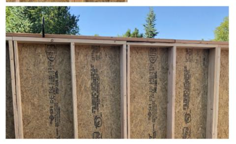
Install top plate on all four elevations. Top plate should be flush with top of wall panel.
